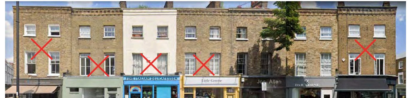
52, 50, 48, 46, 44, 42, 40 Cross Street, Mismatched new windows replace all with double glazed 44 and 42 are correct decorative Victorian type
