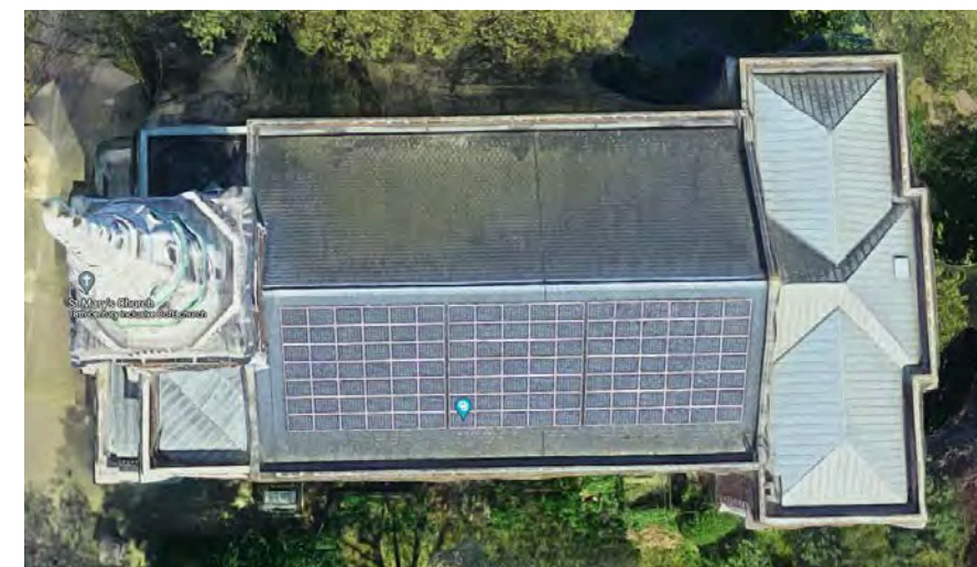
119 panels on St Mary's Church Upper Street
