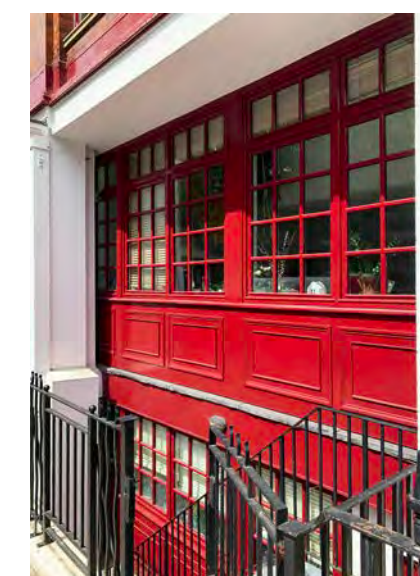
30 Cross St, Recessed Basement window wall. Heritage correct. Double glazed units in old mullions.
