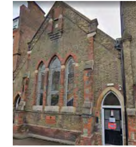
12 Fowler Street secondary glazing
