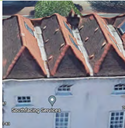
M pantiled roof. Ridge perpendicular to facade
