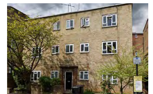
Negative building across Halton street 157
