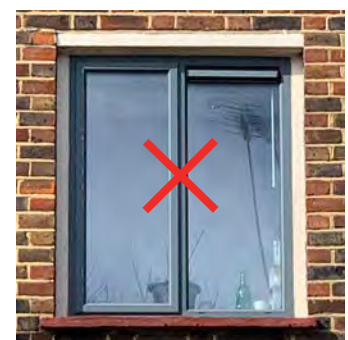
Nearby Florence Street same building above, replaced vinyl
