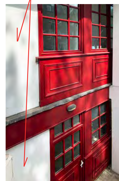
30 Cross St, Recessed Basement window wall. Heritage correct. Double glazed units in old mullions.
