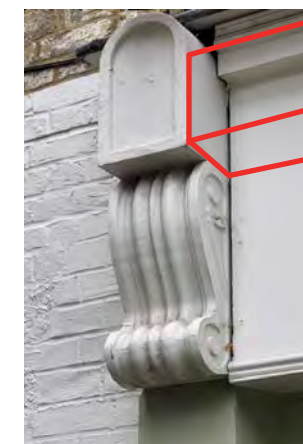
47 Cross Street, Fascia too large, Cornice not aligned with Bracket, bad detail top gaps.
