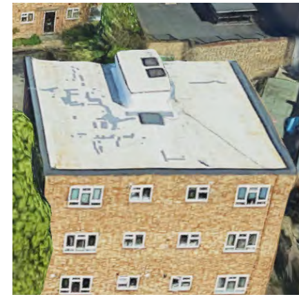
Modern Membrane Flat roofs.
