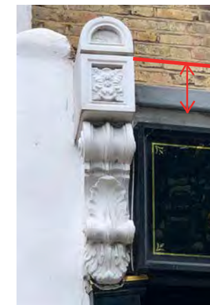
93 Essex Road, cornice
