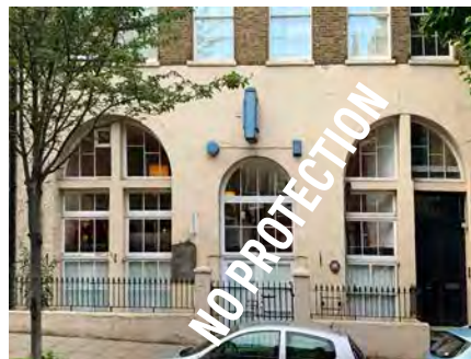
20 Cross Street, new Windows paint dark colour see 30 & 24.
