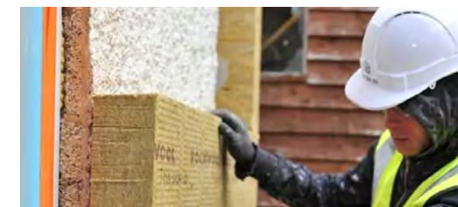
Mineral wool External Wall Insulation install.
