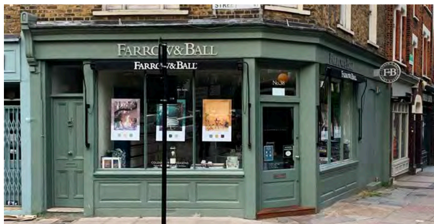
38 Cross St, Heritage correct ready for double glazed windows.
