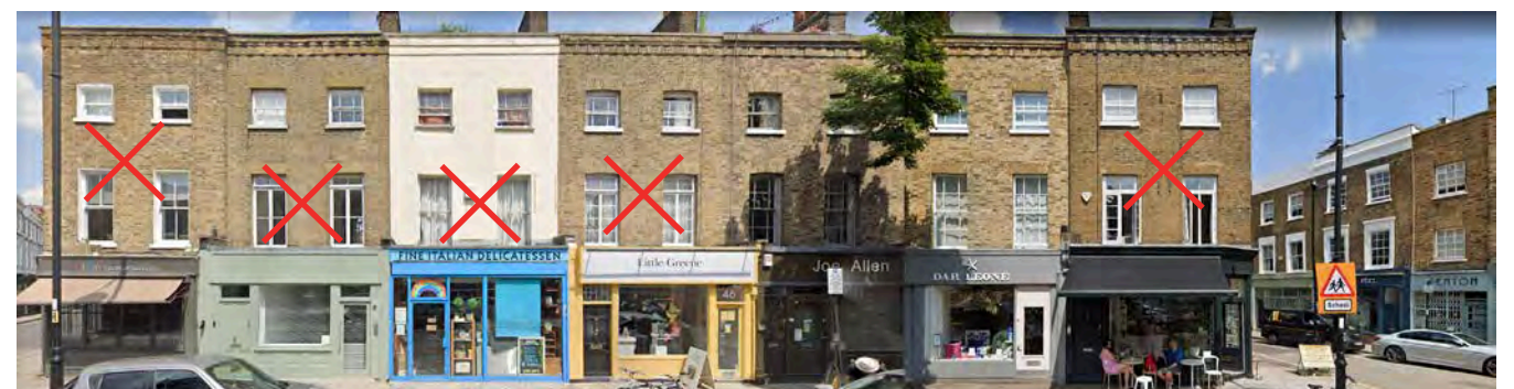
52, 50, 48, 46, 44, 42 Cross Street, Mismatched windows suitable for double glazed replacements
