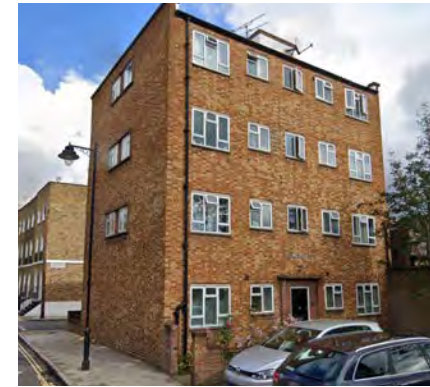
1-8 Fircroft House, Halton Rd Poor finishes, PVC windows, and out of scale, suitable for external insulation, new windows, and balcony/ facade extension.
