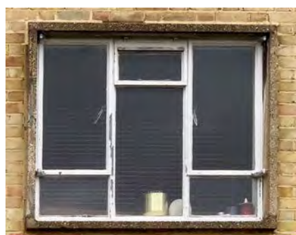
Nearby across Essex Road
