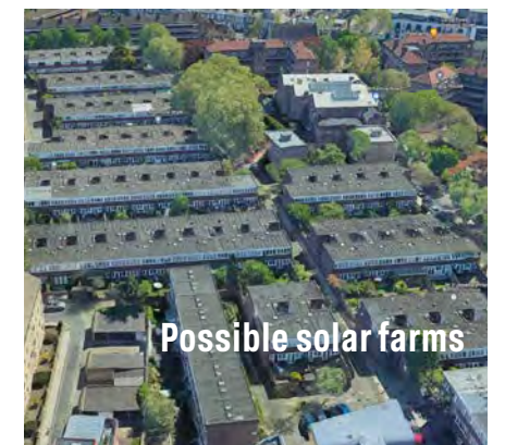
Multiple flat roofs potential Solar farm on council estate
