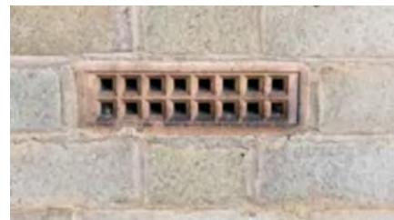
Cross Street - New build
