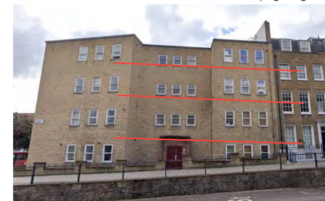
1-8 Belmont House, Cross Street Poor windows, details, and facade composition out of alignment with Heritage Terrace. Suitable for external insulation, new windows, and facade details.
