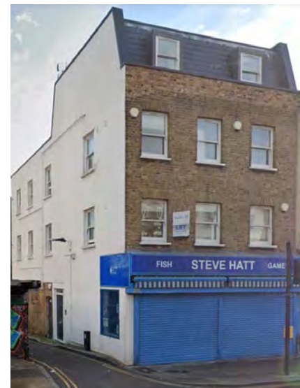
88 Essex Road Modern rebuild lacking historic details suitable for external insulation.
