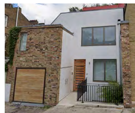
27 Florence Street "Developer Modern" suitable for external insulation.
