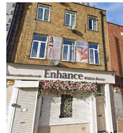
61 Essex Road Modern rebuild lacking historic details suitable for external insulation and new windows.
