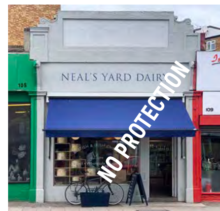
107 Essex Rd, a Unique Parade Pilasters & Brackets should be painted single colour, not split.
