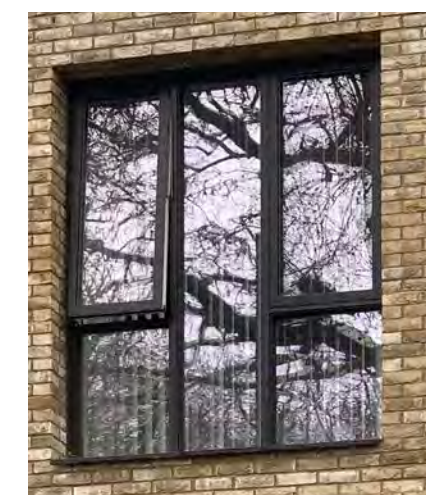
Building nearby outside CA
