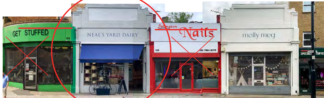
105 Essex Rd, Large signage hiding fascia 107 Essex Rd, Heritage Correct 109 Essex Rd, Large signage hiding fascia 111 Essex Rd, Brackets missing, ext shutter, & door location
