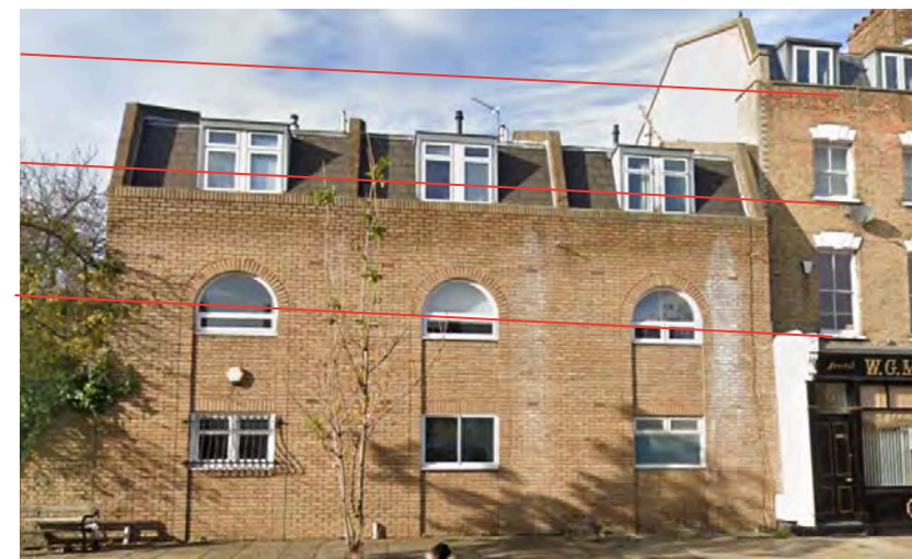
87, 89, 91 Essex Road Out of scale, poor windows and facade, floor heights not matching original terrace . Suitable for external insulation, new windows, and additional storey.
