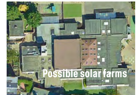
Large flat roofs potential solar farm St Mary's Primary
