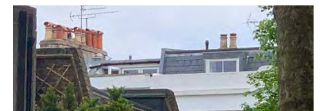
21 & 20 -long view show differing roof heights
