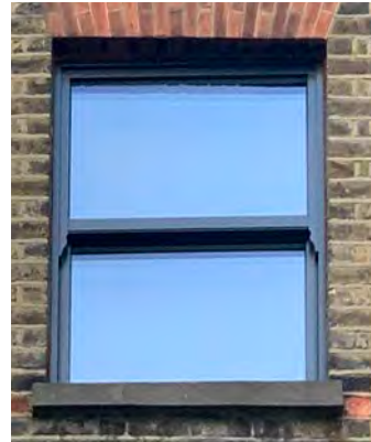
Triple glazed simulated hung sash designed for conservation areas
