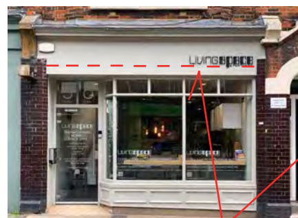
36 Cross St, Fascia covers recessed grill- see 34 Cross St
