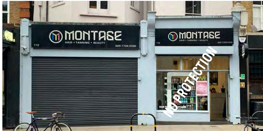
112 & 110 Essex Road, Signage out of scale, Roller shutters
