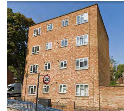
9-16 Fircroft House, Halton Road Poor finishes, PVC windows, and out of scale, suitable for external insulation, new windows, and balcony/ facade extension.
