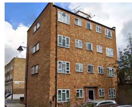
1-8 Fircroft House, Halton Rd Poor finishes, PVC windows, and out of scale, suitable for external insulation, new windows, and balcony/ facade extension.
