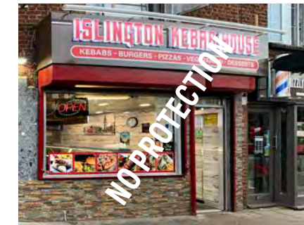
63 Essex Road, roller shutter sign obstructs cornice fascia
