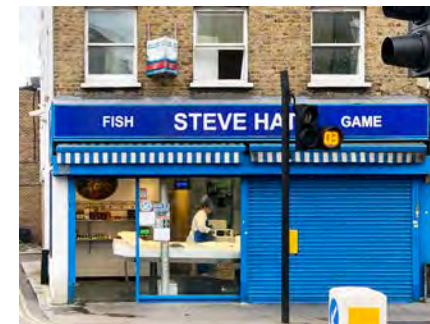
88 Essex Road, roller shutter no stall riser, brackets, cornice.
