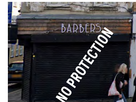
78 Essex Road, roller shutter, sign obstructs cornice fascia
