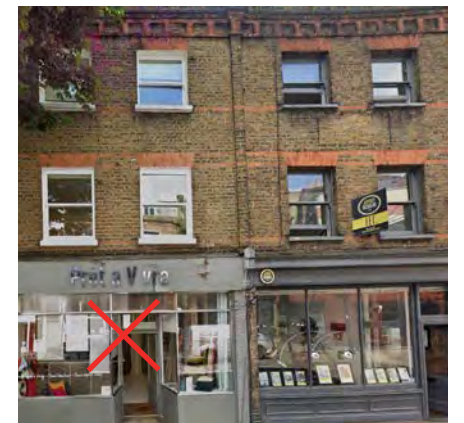
69, 71 Cross Street Shopfront harmed, suitable for Mansard fill in
