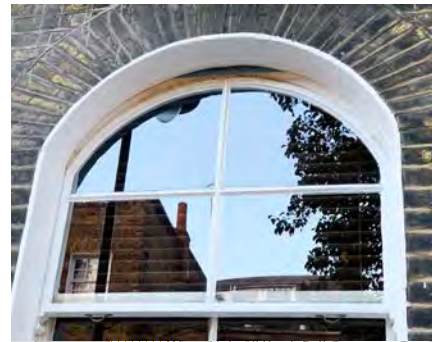
Correct timber slim-profile double glazed slim -profile, Halton Road
