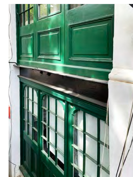
24 Cross St, Basement recess.
