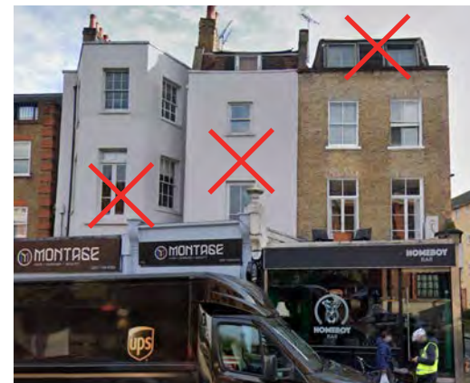
112, 110, 108 Essex Road Shopfronts harmed, new windows mismatched with reduced size. Suitable for external insulation & windows.
