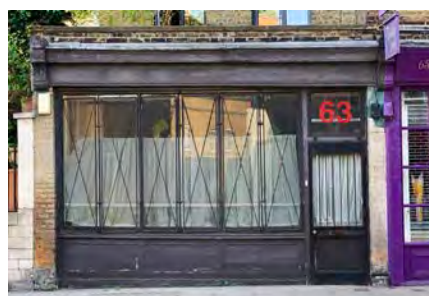
63 Cross St, House,return Shop, replace grills for a better street
