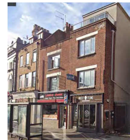
63, 65 Essex Road Poor windows and building massing at roof level suitable for external insulation and new windows
