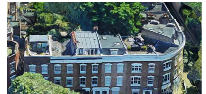
Google 2022, ©The GeoInformation Group 2022 23, 21, 20 & 17 Dagmar Street Extensions
