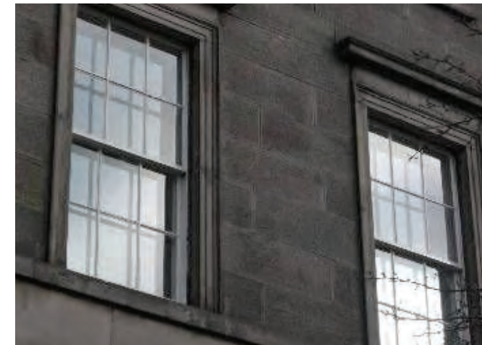
Secondary window visual impact of reflections on inner secondary windows harms heritage in Conservation Area. Research found by the trial installation of different double glazed unit types in Edinburgh Georgian tenements, by the Changeworks project mentioned above. 2
