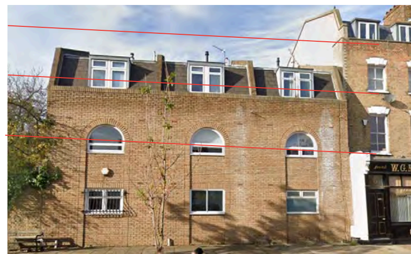
87, 89, 91 Essex Road Out of scale, poor windows and facade, floor heights not matching original terrace. Suitable for external insulation, new windows, and an additional storey.
