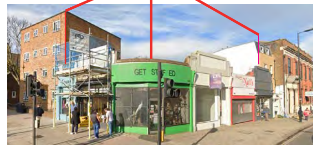
6 shop parade Cross & Essex. Shop fascia and windows damaged, Positive heritage fascia to retain.
