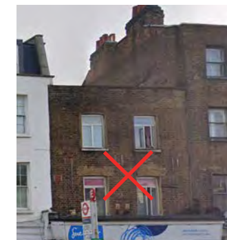
72 Essex Road casement windows damage heritage, suit 2 over 2 sash triple glazed.
