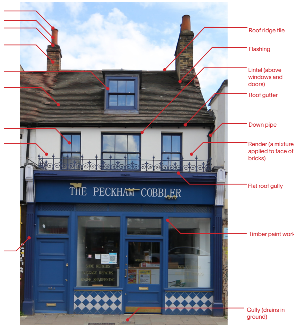
Image: 102 Peckham High Street after works in 2021
