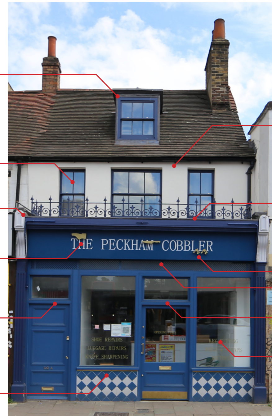
Image: 102 Peckham High Street after works in 2021
