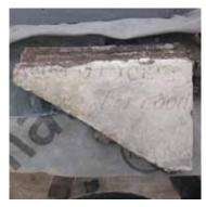
process of removing the coping stones, it exposed Victorian costing cutting approaches, using graveyard artefacts. The roof covering was extensively repaired and upgraded with new slate tales, lead flashing and the upper cornice was repaired by implementation of the technique of applying successive thin layers of render of ever sharper definition using a "horsed" mould run on levelled rails.
