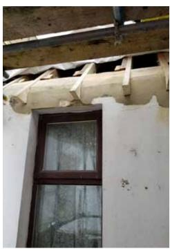
The recent condition to keep the building functioning had been entirely pragmatic and utilitarian. As a result, we addressed releveling the adjusted eaves level surface water drainage from the roof, the reinstatment of the dormer and timber pilaster heads, redecoration of the cement render, complete overhaul of the projecting roof top and drainage.
